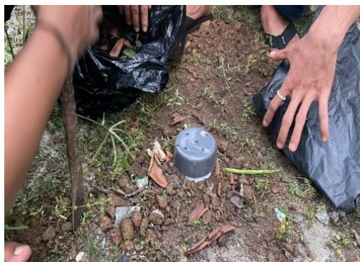
Gambar 2. Penanaman Pipa Biopori
